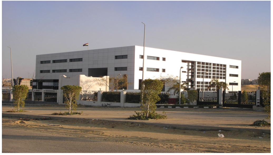
Administration Building For PGESCO Co . ( New Cairo City )
