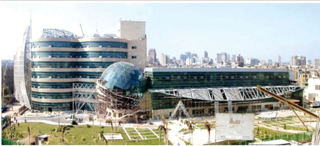
Front Facade - Children's Hospital ( 57357 )
